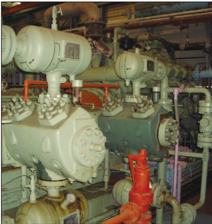
■ This Ingersoll Rand RDH compressor is driven by a Waukesha L7042 GU natural gas-fueled engine. The compressor is a four-throw, four-cylinder unit that uses four stages of compression to achieve a delivery pressure of 900 psig (62 bar) for sweet gas or 1100 psig (76 bar) for sour gas.
