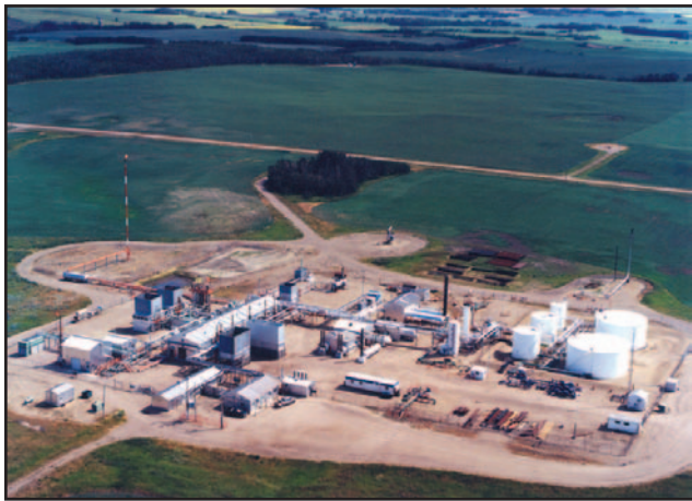
■ The Clive area is located in central Alberta, Canada, approximately 30 mi. (50 km) northeast of Red Deer. Fairborne Energy Trust operates this oil processing and gas compression facility, which handles up to 16,500 bbl/d (2625 m 3 /d) of crude oil and 25 MMscfd (7.1 x 10 5 m 3 /d) of natural gas. This photo was taken before modifications to the plant commenced.
