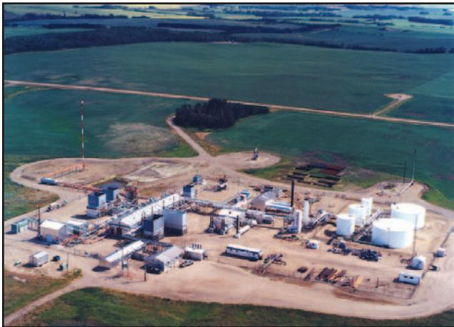
■ The Clive area is located in central Alberta, Canada, approximately 30 mi. (50 km) northeast of Red Deer. Fairborne Energy Trust operates this oil processing and gas compression facility, which handles up to 16,500 bbl/d (2625 m<sup>3</sup>/d) of crude oil and 25 MMscfd (7.1 x 10<sup>5</sup> m<sup>3</sup>/d) of natural gas. This photo was taken before modifications to the plant commenced.
