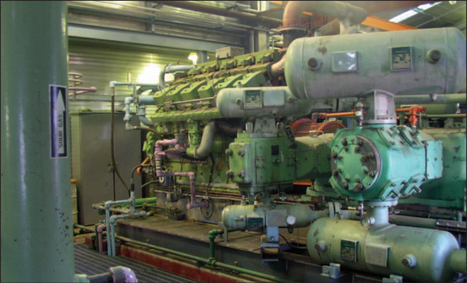
■ Unit C308 includes a Clark CFB compressor and a 604 hp (450 kW) Waukesha L5108 GU engine. This gas processing facility has been designed to use large compressors with low-pressure capabilities, and as such, the first stage of compression requires very large 24 in. (609.6 mm) cylinders.
