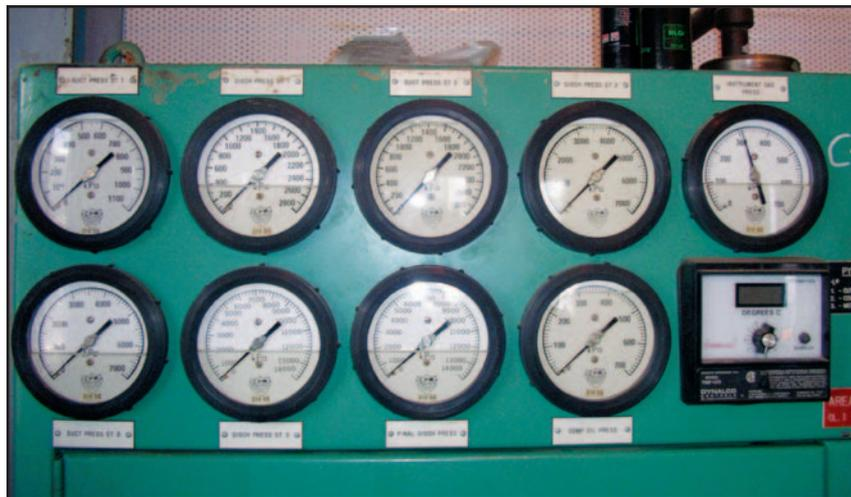
■ This compressor plant is operated manually. Each compressor has its own control system to monitor its operation, including speed control and safety shutdown. The control systems are independent and mainly pneumatic.
