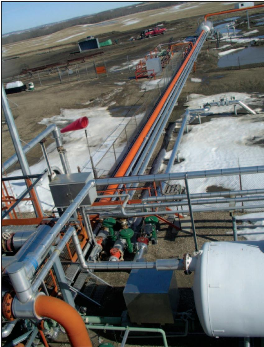
■ The gas compression facilities were constructed using the California model of the '40s, '50s and '60s. One feature of that design is the location of the auxiliary equipment, such as the coolers, filters, scrubbers and dehydrators, which are far away from the compressors.
